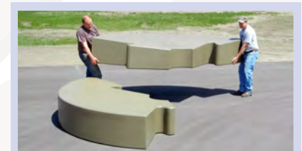
Installing cone bottom design
